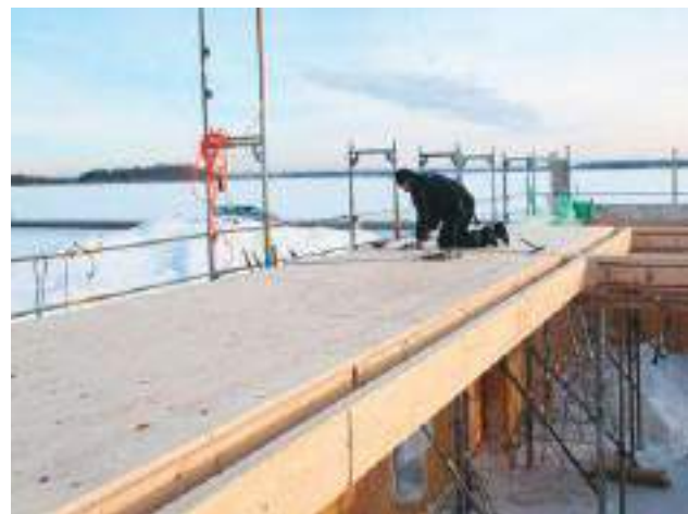
STEICO LVL X as a stiffening decking element for pre-assembled floor cassettes
