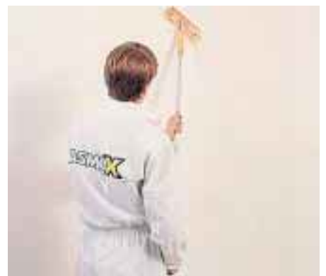
Fillers adhere to the gypsum surface of the board readily. Any dust and other impurities on the board surface should be removed before surface coating the board.
