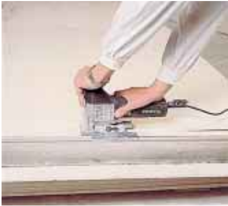
A jig saw can also be used without the suction unit to produce different - even complicated - cuts on the panel.
