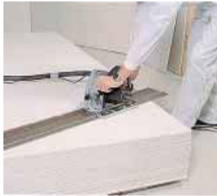
Using a hard-metal circular saw and a guide rail to enable fast and safe sawing of the boards. Narrow strips can be sawn with the board resting on the stack.
