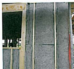
Below: the timber frame is filled with Thermo-fleece sheep's wool insulation
