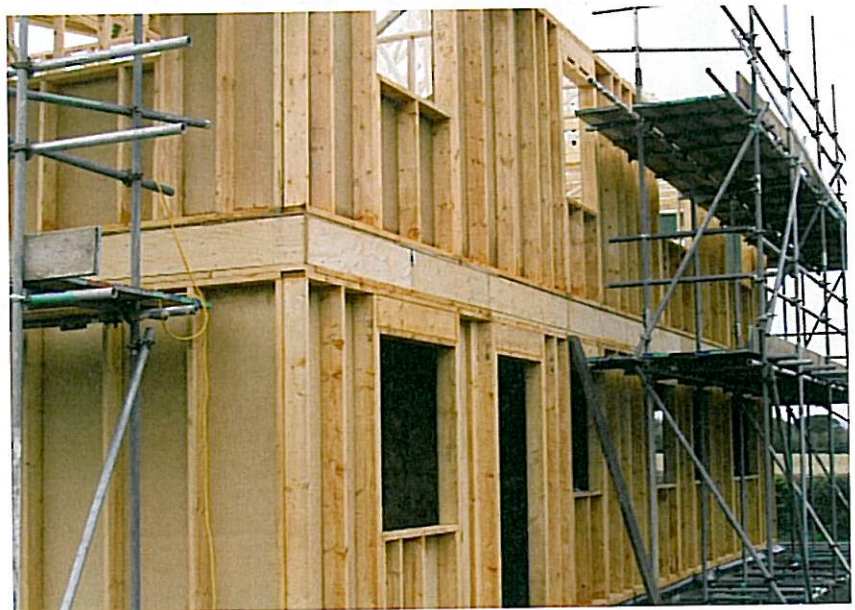
Above left: glulam feature beams
