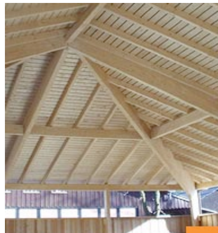
Glulam in a roof application
